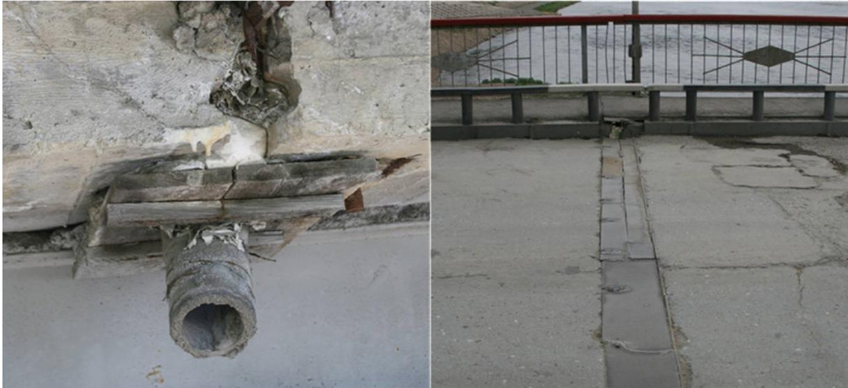
*Fig. 2. Drainage pipe (left) and expansion joint (right)*
